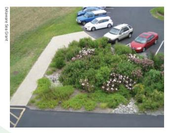
Green infrastructure is used to reduce flooding.
