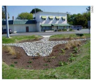
Vegetated swales are a nature-based technique to manage stormwater runoff.
