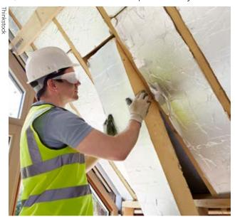
A weatherization professional installs insulation panels into the roof of a home.
